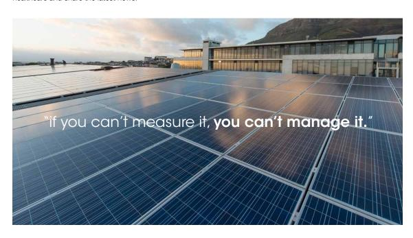
We put in a 400 kWp solar PV system, comprising 1 298 modules over a rooftop area of 2 519 m<sup>2</sup>, at our head office building in this financial year.
